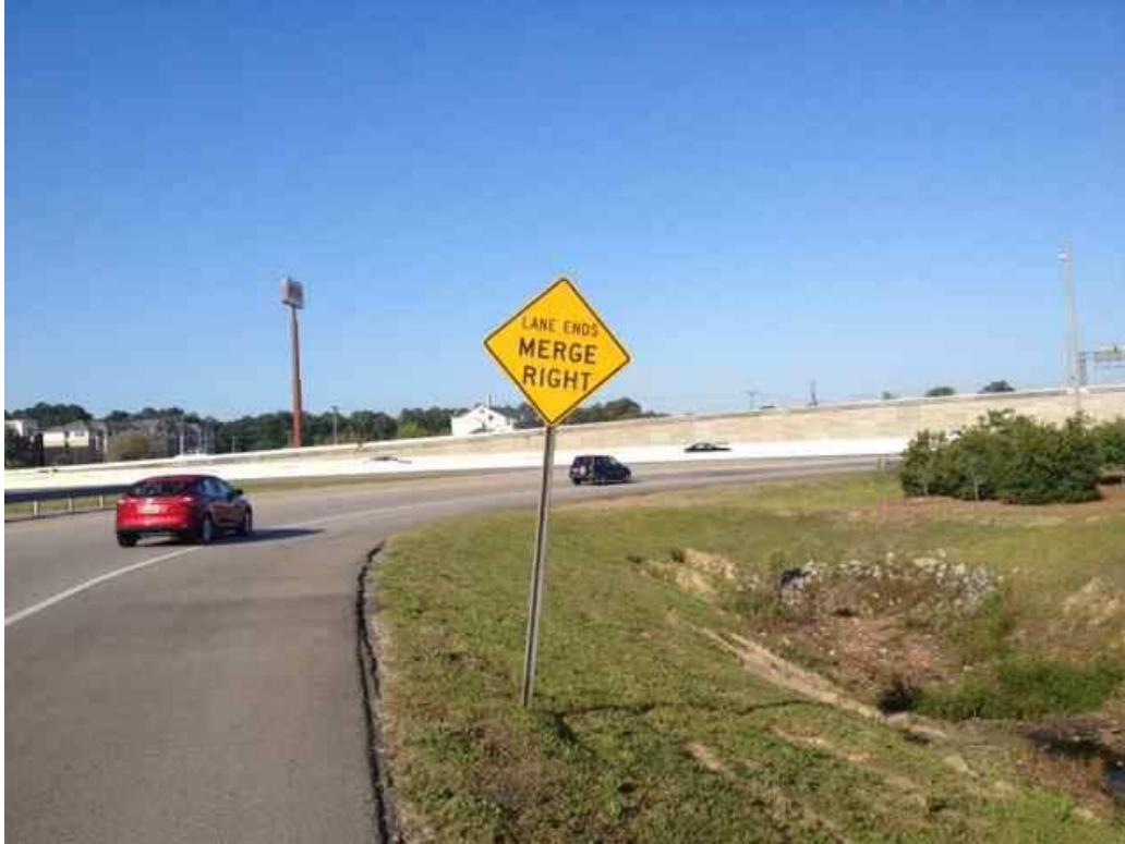
Photo 1: Ramp, just prior to entry onto the interstate ramp.
